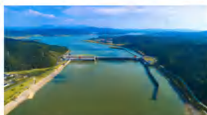
Hydrological and Water Conservancy Monitoring Platform
