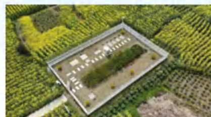
Rural Sewage Monitoring Platform
